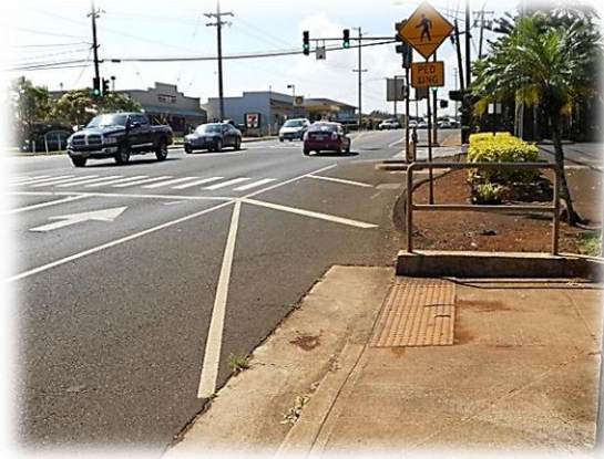
Pictured above: Hanamaulu/Kuhio Hwy sidewalk end
